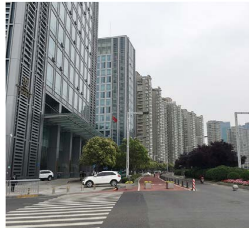
▲ Over 80% of the total existing office stock in Zhengzhou was sold "strata-title." Source: JLL Research
